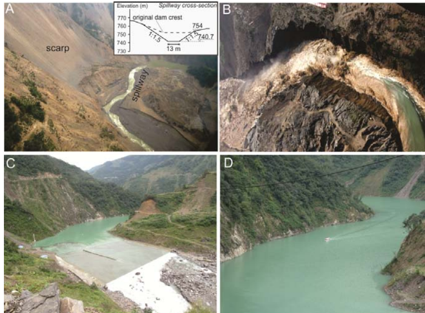
Figure 7.5 A: Helicopter view of the artificial spillway, inset shows the spillway cross-section; B: Releasing impounded water through the spillway, taken on June 10, 2008 when the discharge reached its peak (provided by Dr.Liu, N. from Ministry of Water Resources of the People’s Republic of China); C: Remaining dam; D: Remaining lake, C and D were field photo taken in Sep, 2011.
