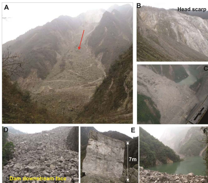
Figure 2.9 Laoyingyan landslide. A: Overview of the Laoyingyan landslide; B: Head scarp; C: Helicopter view of the dam body; D: Dam downstream face; E: The largest boulder in the deposition zone; and F: Barrier lake.
